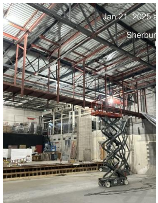
Diamond Plate install on Catwalk
