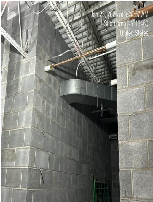
Ductwork Installation In New Walls
