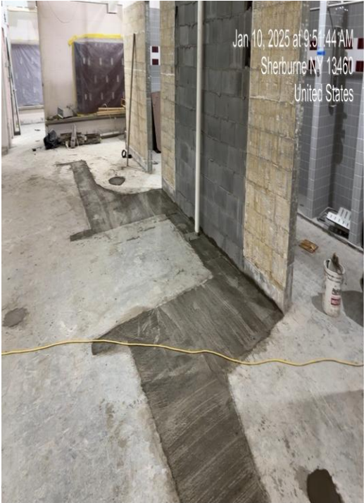
North Locker Room Concrete Floor Infills
