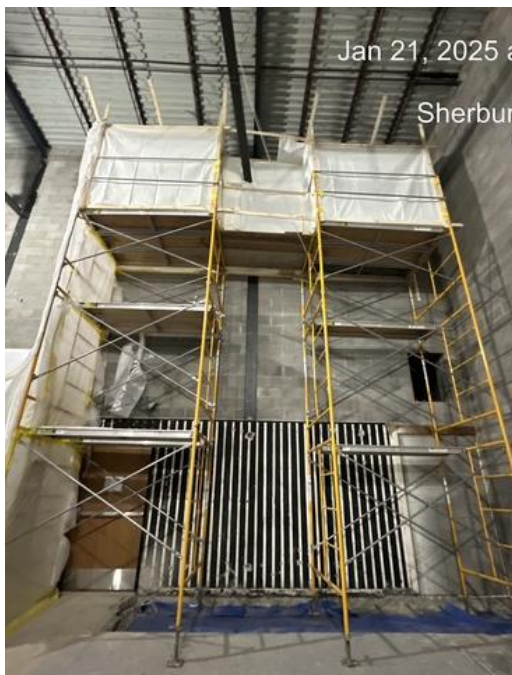
Abatement Decon for Duct Penetrations
