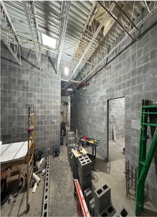
ATL Onsite for Concrete Testing
