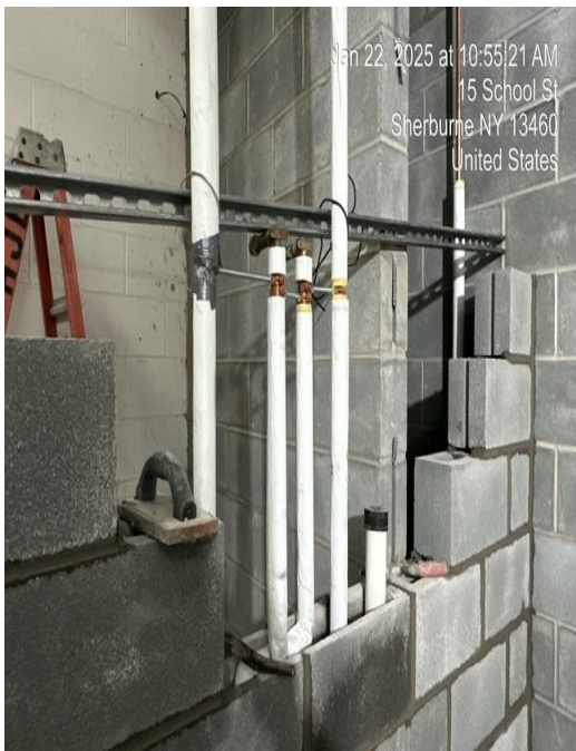
Plumbing Rough Ins
