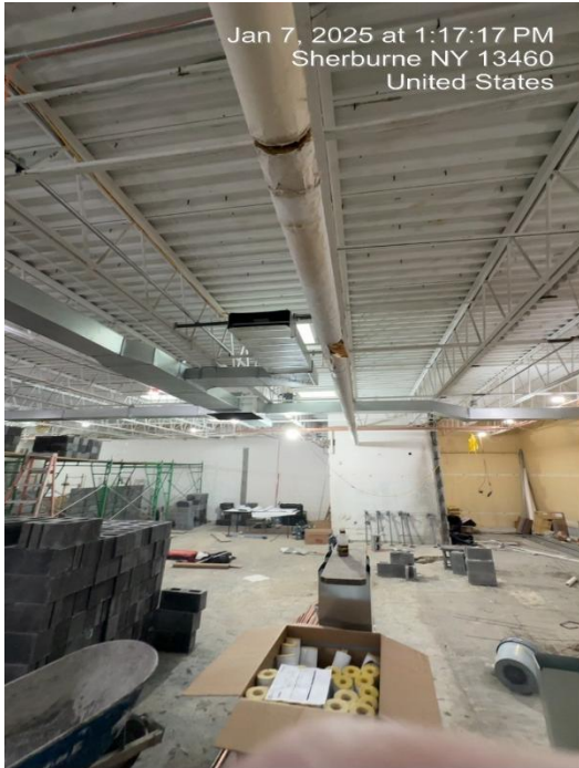
2" Heating Line removed for relocation
