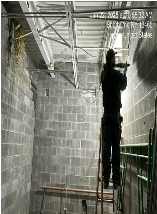
Cutting in for Transfer Grilles
