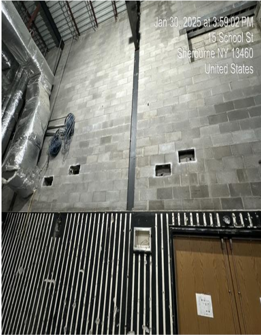
South Wall Penetrations
