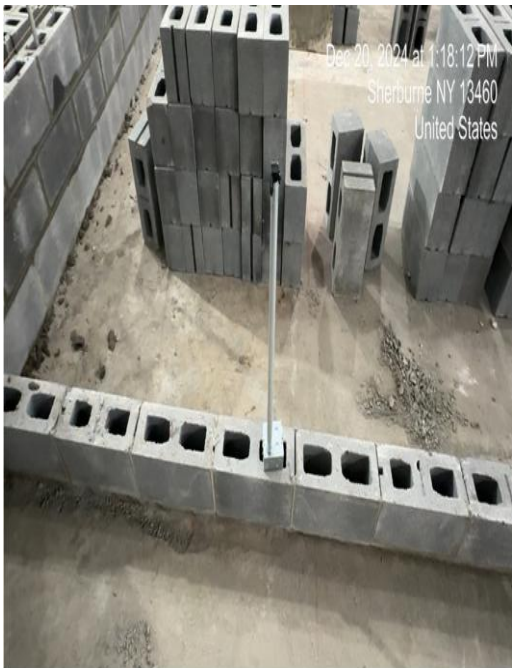
Electrical Rough Ins in New CMU Walls
