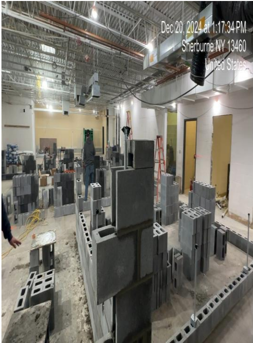
CMU Wall Layout in South Locker Room
