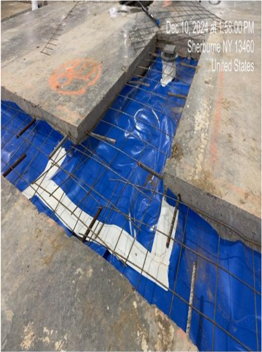
Rebar and Wire Mesh Installations in Slab Cut Outs
