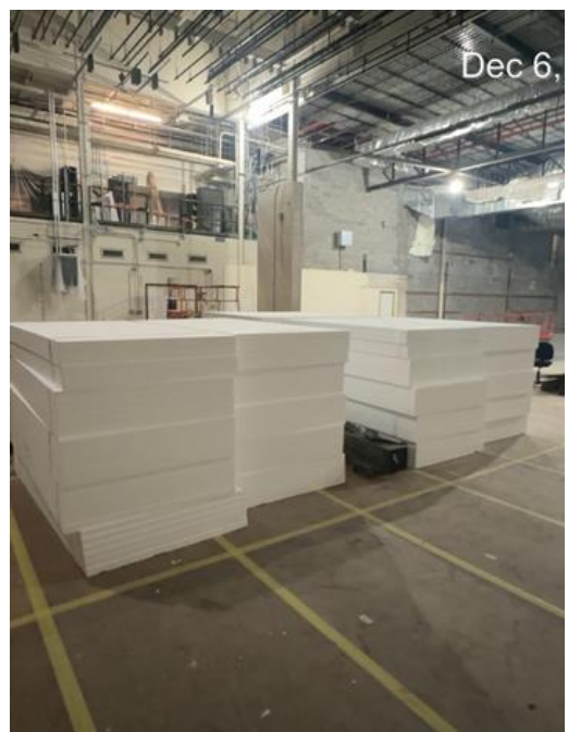
Concrete Slab Geo-Foam Delivery
