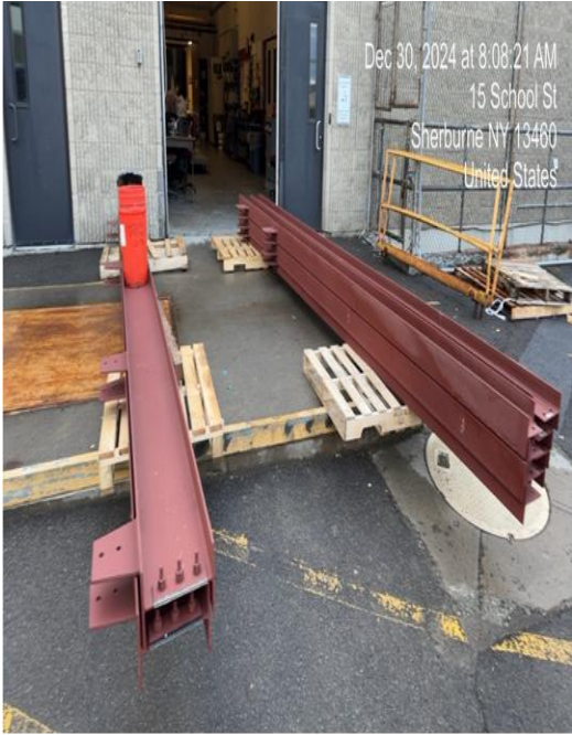
Catwalk Structural Steel Delivery
