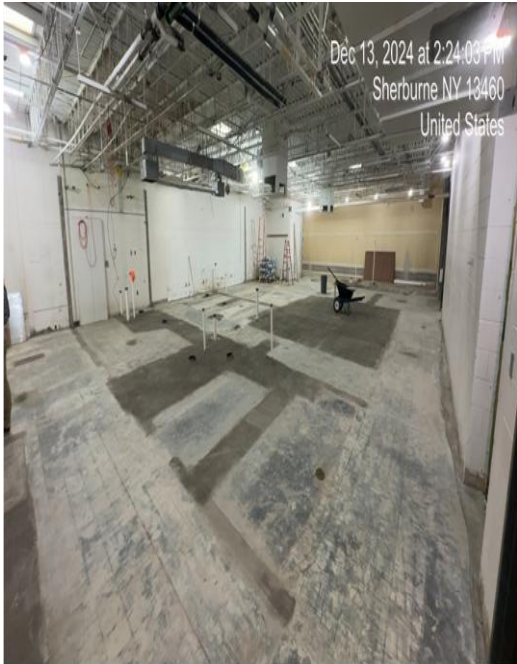
Concrete Floor Infills Completed
