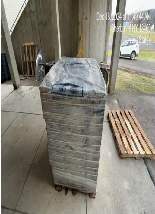
Mortar Delivery for New CMU Walls
