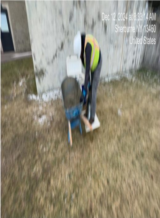
ATL Onsite for Concrete Testing
