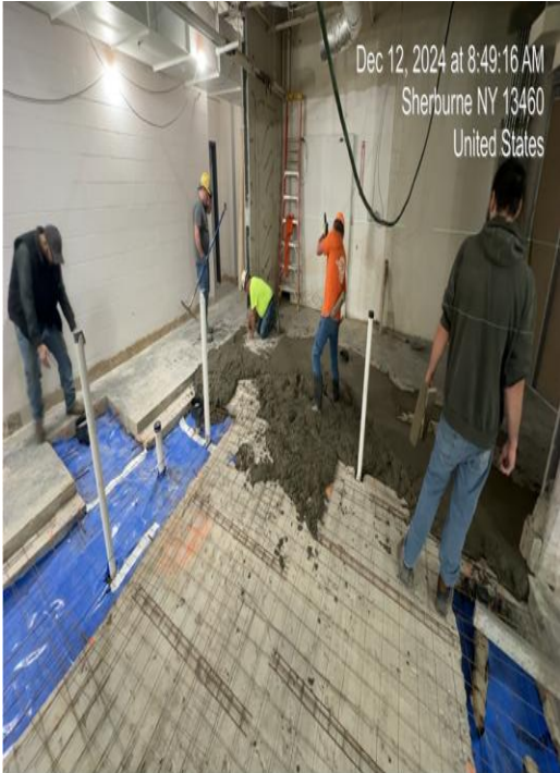
South Locker Room Concrete Floor Infills
