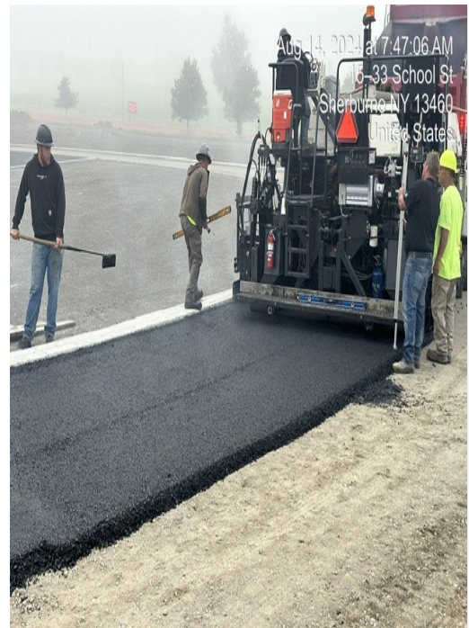
Track Asphalt Paving Began
