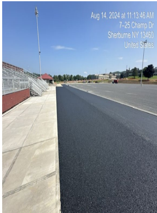
Top Course Asphalt Paving
