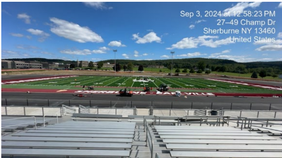
Current View of Construction
