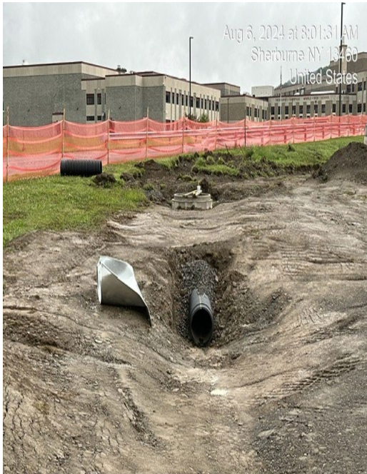
Stormwater Drainage Installation
