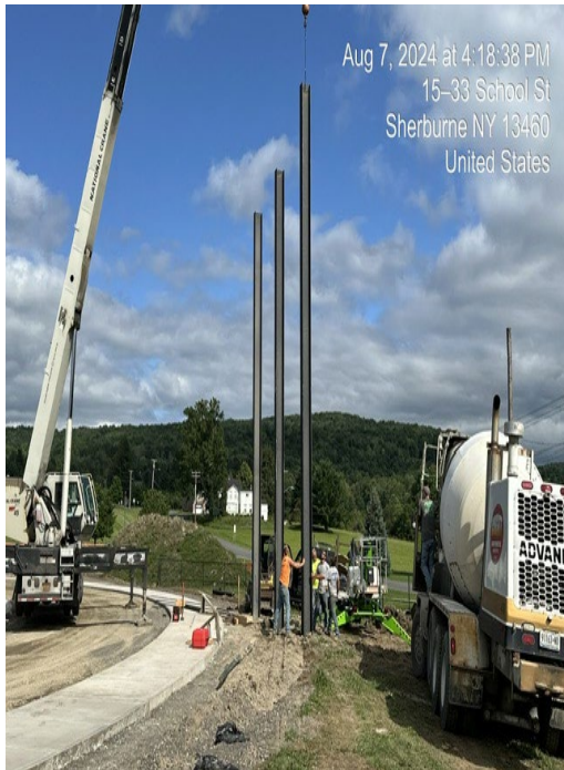
New Scoreboard Steel I-Beams
