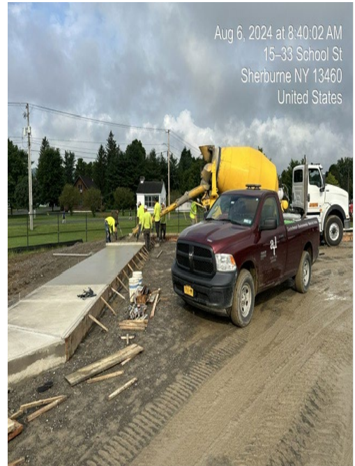
ATL On-site Testing Concrete
