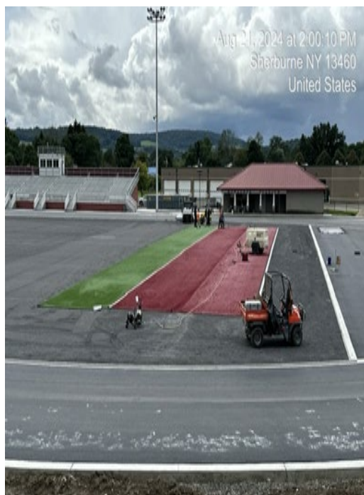
Turf Install Begins
