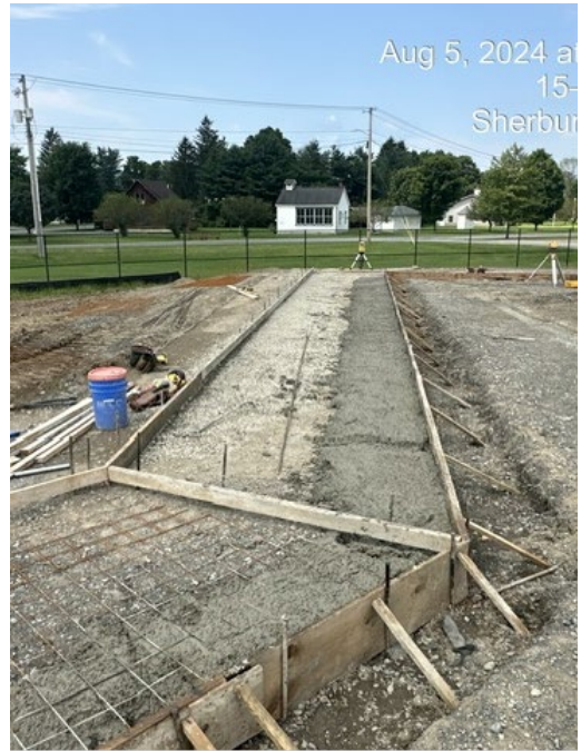
Concrete Sidewalk Forms and Reinforcement
