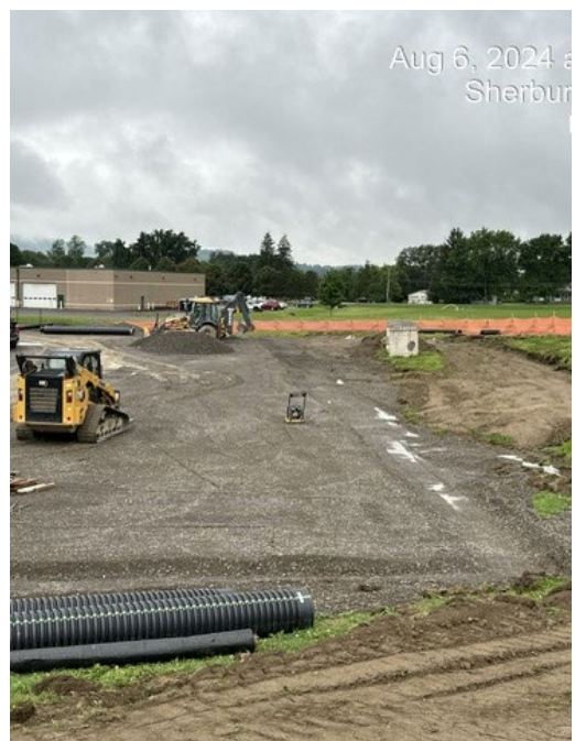
Final Subgrade Grading
