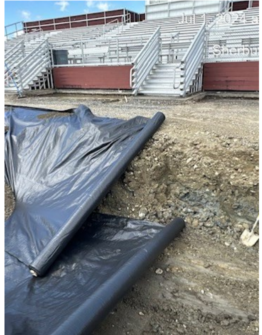
Stablization Frabric in Track Subgrade Cuts
