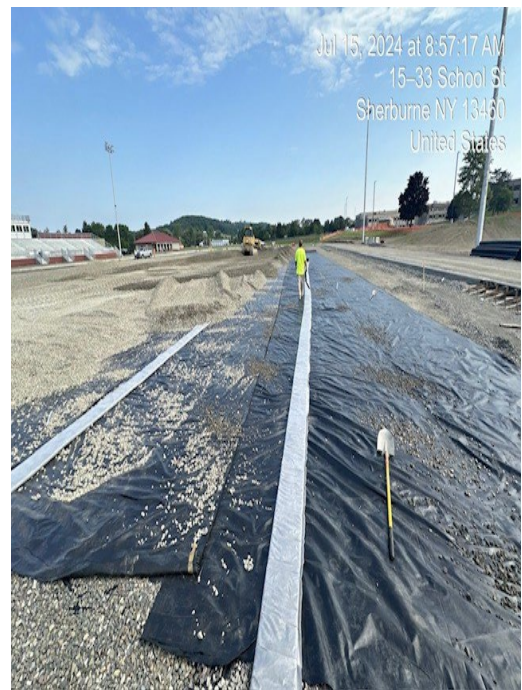
Field Fabric, Flat Drain, and Subbase Stone Install
