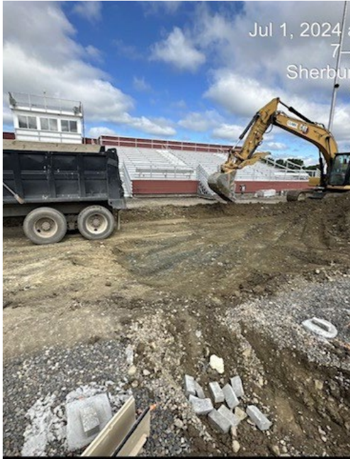
Track Subgrade Material Cut Out
