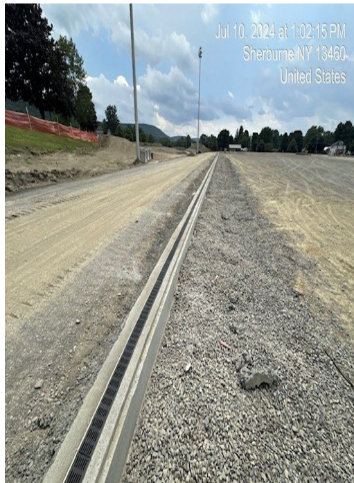
Finished Perimeter Slot Train
