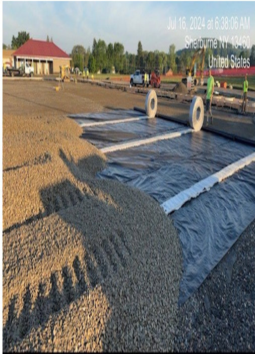
Extra Section of Flat Drain
