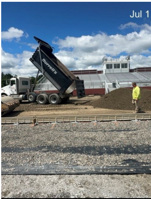
Track Subgrade Soft Areas filled with Item 4
